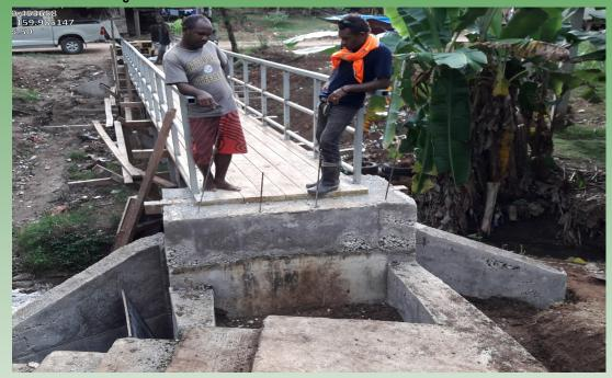
Milestone footbridge is in the final stage of completion. Last week the contractors put up the flooring and rails. Currently contractors are doing back filling and final touch then the footbridge is ready for use. Already the community are excited of their gift.
