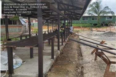
Concrete slabbing and construction of market tables and benches in Munda market has been completed. Currently the local workers are working on the drainage system. As soon materials are ready for the other buildings then work will kick off immediately.
