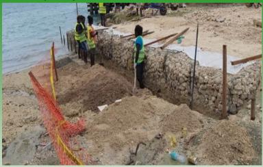
The Munda jetty is progressing very well at the moment although work has been affected by the continuous bad weather in Western Province. At present community workers are working hard filling up the gabion basket with stones and aliening them to their designate areas ahead of the construction of jetty. Titus Maina; Resident Works Supervisor in Noro said work according to the speed of work taken by the community workers we expect to complete the jetty according to the time frame.
