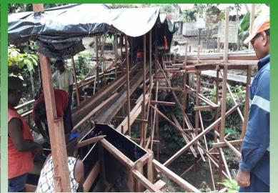
Botanical footbridge has reached the footing stage. Currently the local workers are working on aligning the beam to follow by flooring and railing. The project is aim to complete next month.
