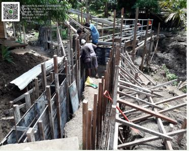
Work on the new footbridge at Antioch in the Central Honiara is progressing very well at moment. Currently the workers are working on foam works and structures of the bridge before actual pouring of concrete will take place in the coming weeks.
