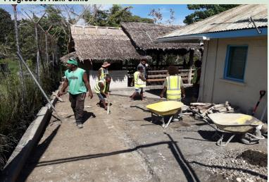
Work on slabbing the Auki clinic Ablution block is progressing very well at the moment. Currently local workers are working on drainage system and payment of the clinic. This will address flow of water system and protect the clinic surroundings.
