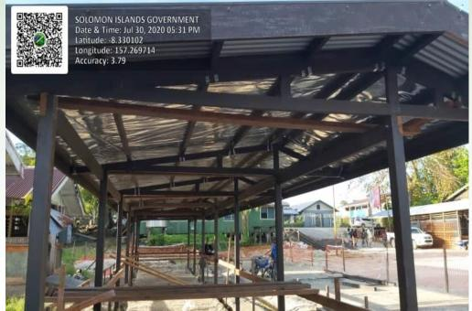
Work on Munda New Zealand funded market building is progressing very well. The roofing on the building has been installed.
