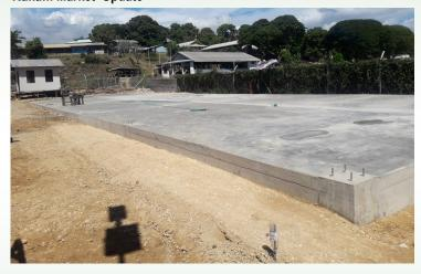
The construction of Kukum market is progressing well with the slabbing of basement. Procurement of materials for CAUSE contribution into the project is well taken care of. Work is progressing well and we should be able to fill in our part to the project pretty soon. The market once completed it will be a facelift to Kukum resident but also the main source of local food to the eastern side of Honiara.
