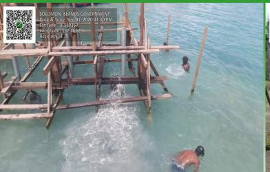
The construction of Munda jetty is progressing very well. This week the local workers are working on displacing underwater sand for concrete placement. As soon as the concrete are dry they will start work on the flooring of the jetty.
