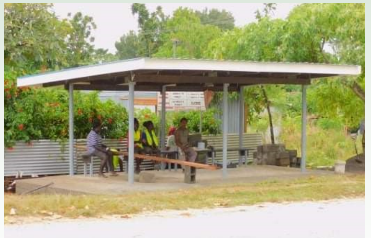
The newly built busstop at Noro has been completed. The new busstop is located in front of the Solomon power staff quarters at Noro. Residents who resided along the Baru area thanked and acknowledged CAUSE project for the shelter.
