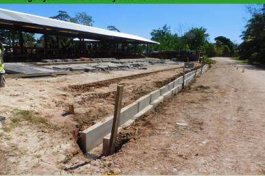
Drainage system on the Banana valley satellite market in Gizo is progressing well. Currently there are number of culverts in position to be burry. The area is always filled up with water and mud. With the improved drainage system it will give a facelift to the new market.
