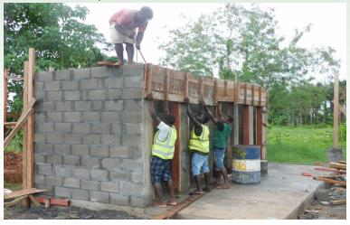
Banana valley satellite market ablution in Gizo is almost in the completion stage. In the coming weeks works will install roofing to be followed by internal works and plastering.
