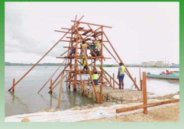
The construction of Noro market jetty has started this week. Currently workers are working on piling structures. In the coming weeks they will be working on aligning the posts and other structures of the jetty.
