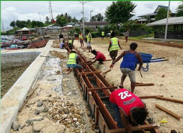
Local workers working on the Noro fish market are currently working on the form work ahead of concrete slabbing over the coming weeks. The aim is to complete the work by mid September.
