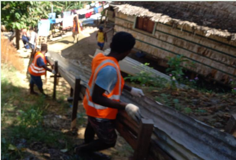
Workers this week align the drive way for concrete pouring ahead of next week. So far all form work has been completed and workers are looking forward for the concrete slabbing.
