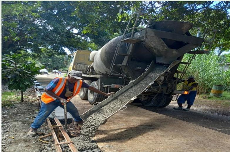
Work is still ongoing for drainage system and lane two of the Vura road. The first concrete and drainage system on the Vura heights has been completed now workers moved to the other side of the community.
