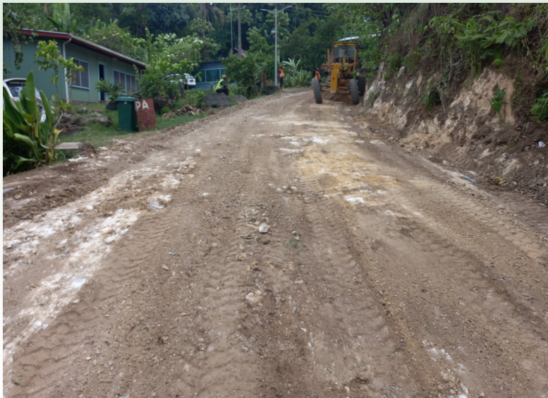
Grading on Lai's road at Mbokavera 3.
