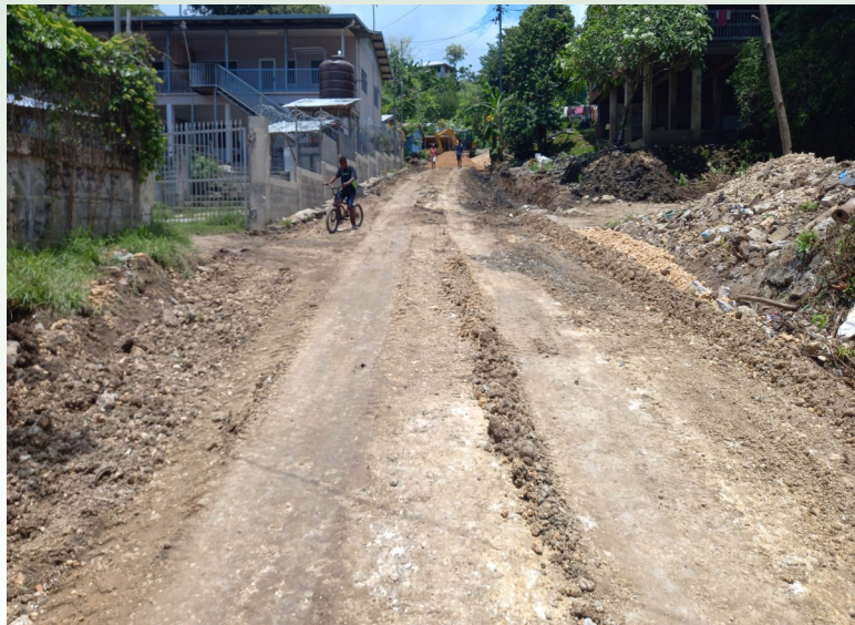
Compacting of Adams road at Mbokanavera 1 ahead of concrete works.
