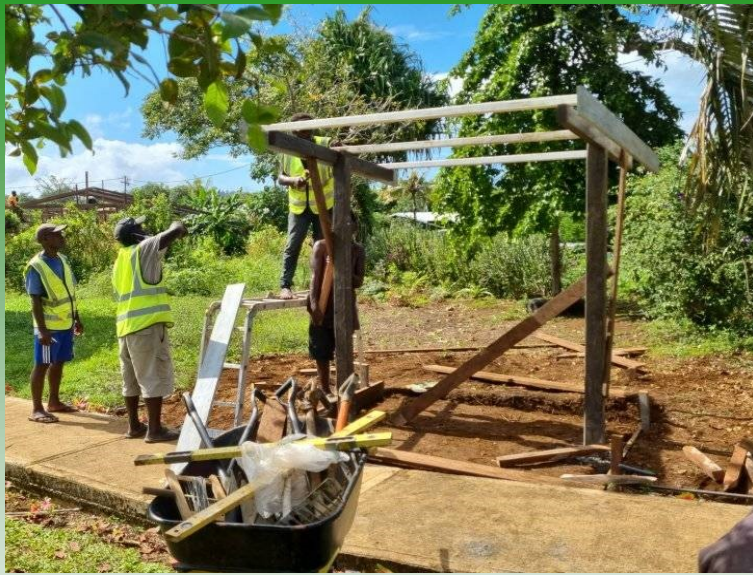
Noro team is currently working on installation of wash bay stations for schools and public spaces in Noro.
