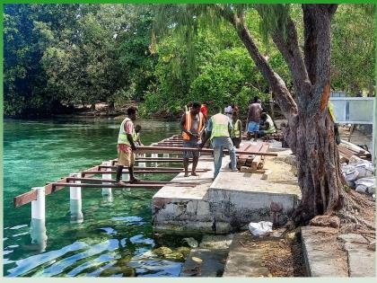
Work on Nusatupe jetty at Gizo has resumed following arrival of timbers on site. Installation of floor joist and decking is going on and is expected to complete in the coming weeks.
