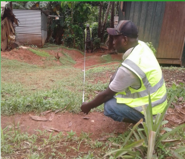
Gizo PIU foreman measuring and conducting pegging work ahead of the construction of a new 100 meter Jacob's ladder at inner banana valley.
