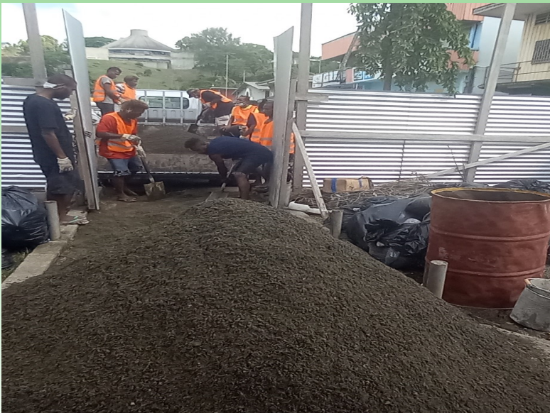
Workers unloading gravels ahead of next weeks brick works
