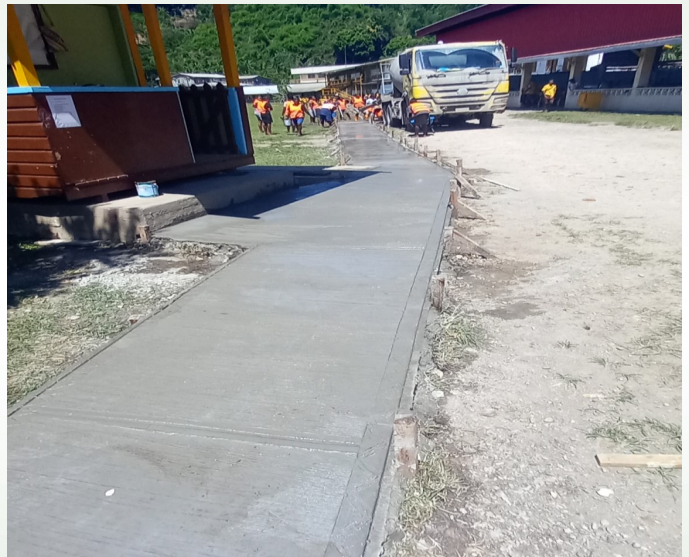
The Honiara High School footpath has completed this week.
